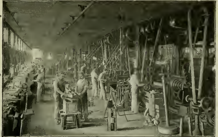
FINISHING CROSSHEADS—BALDWIN'S.
